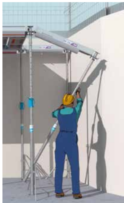
The extendable beams let you go near the cell edges
