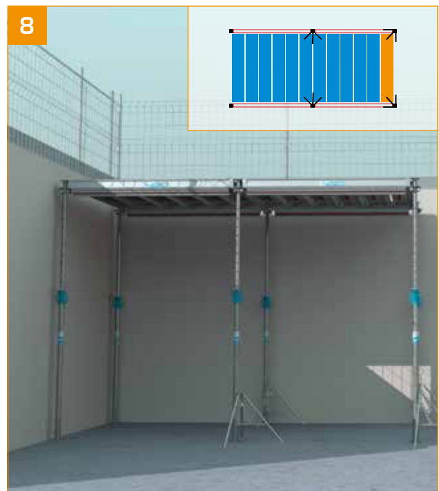
- Repeat steps 5 to 7 and finish installing the Eco+ closest to the wall.
